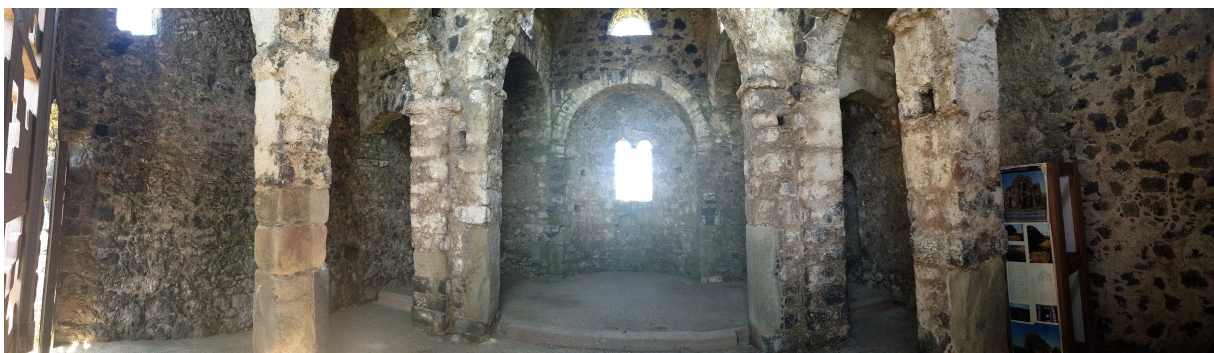
View of the interior of the church (Wikimedia Commons)
